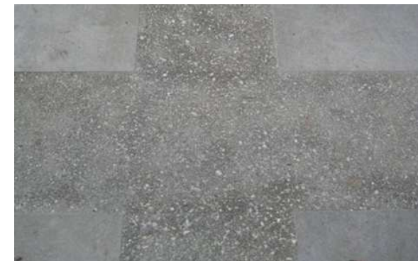
EXAMPLES OF 'ABRASIVE BLAST FINISH (HEAVY) TO TRAM SHAPE. ALLOW FOR LASER CUT STEEL TEMPLATE TO CREATE PATTERN. USE BLACK AGGREGATE SO THAT THE EXPOSED AGGREGATE REPLICATES THE EXISTING BALLAST.'
